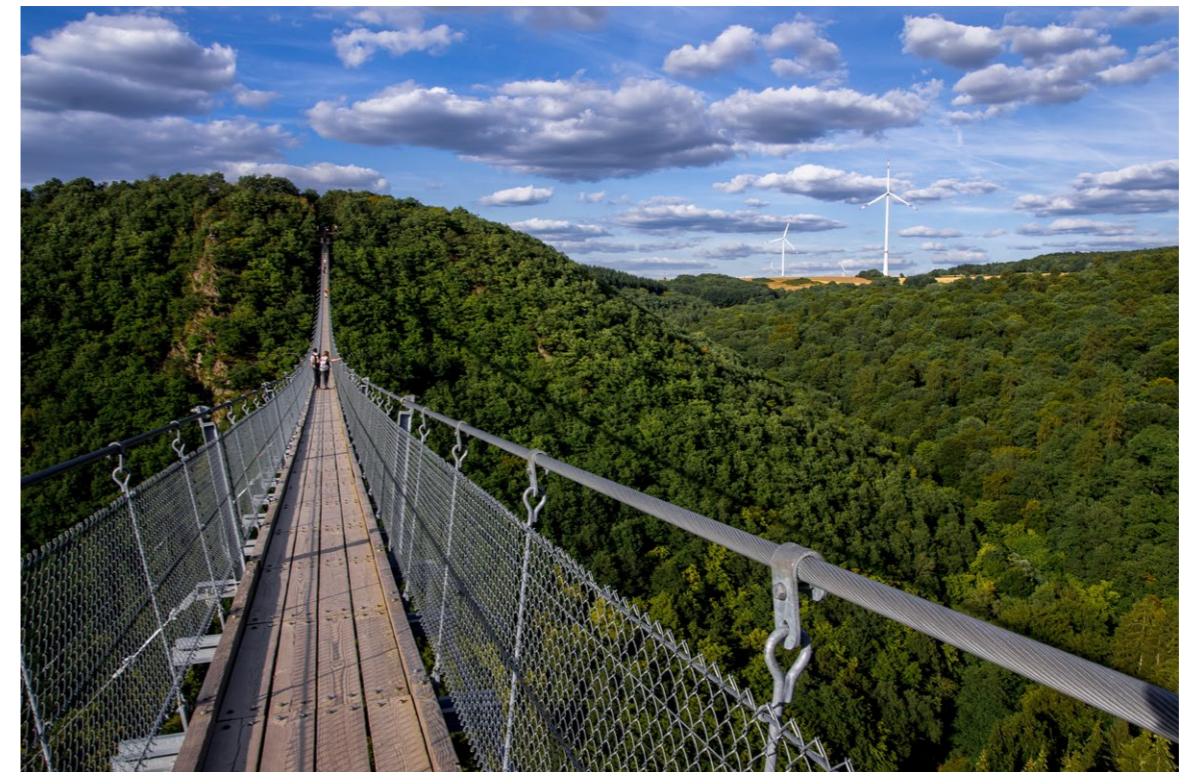
Figure 9 Geierlay Bridge. Source: Gilbert Sopakuwa, CC BY-NC-ND 2.0
