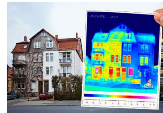
Areas of heat loss are easily identifiable in the thermal image: the uninsulated left half of the house is losing a lot of energy through the facade. The thermal image also clearly shows the weak spots at the windows.
