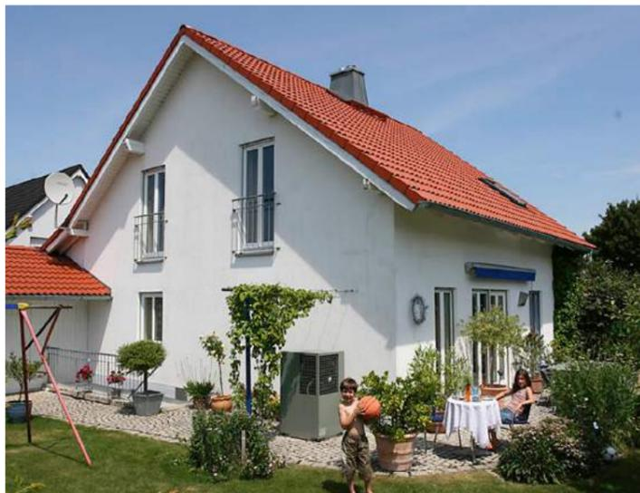
Ambient air can also be used as a heat source for a heat pump located in the garden.
