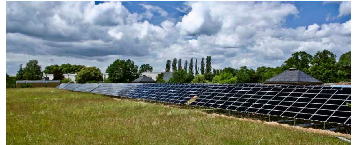
The solar plant on the roof of the underground drinking water cistern in Berlin-Tegel with its areas of protected fresh and dry sandy grassland is a unique biotope. (Photo: First Solar GmbH)
