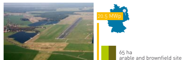
Rothenburg solar park Gehrlicher Solar AG, completed 2007
