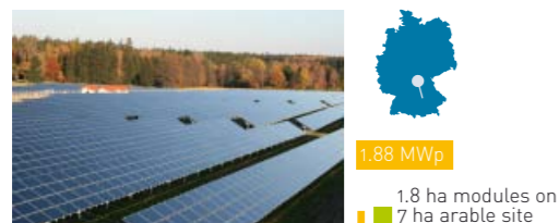
Sulzemoos solar park Phoenix Solar AG, completed 2007
