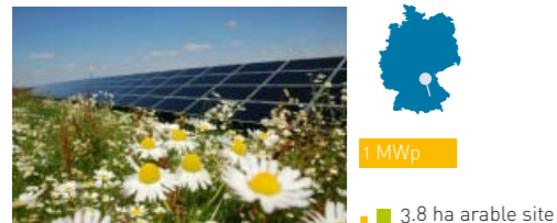
Salmdorf solar park Gehrlicher Solar AG, completed 2007
