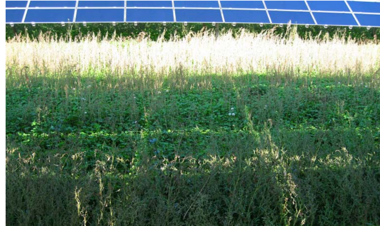
Lush vegetation grows even underneath the modules. Gaps between the modules allow even rainfall. (Photo: BELECTRIC)
