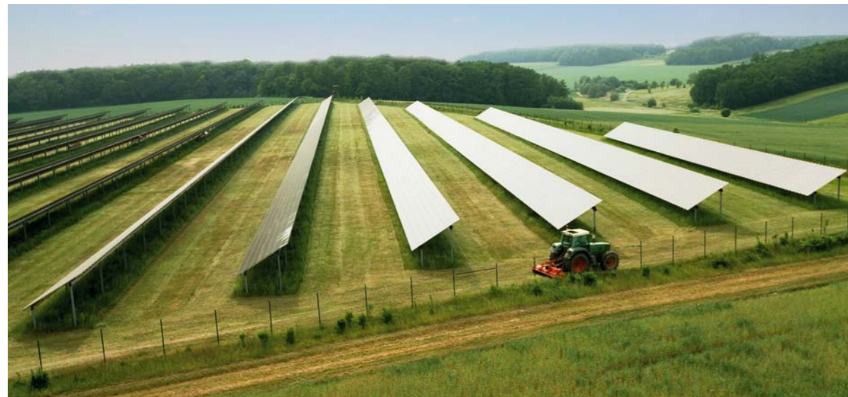
To conserve the open spaces, grassland surrounding the solar plants has to be mown at regular intervals. (Photo: BELECTRIC)
