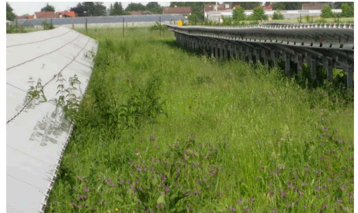
Fences are necessary for security reasons, but should allow enough space for small animals to pass through. (Photo: First Solar GmbH)
